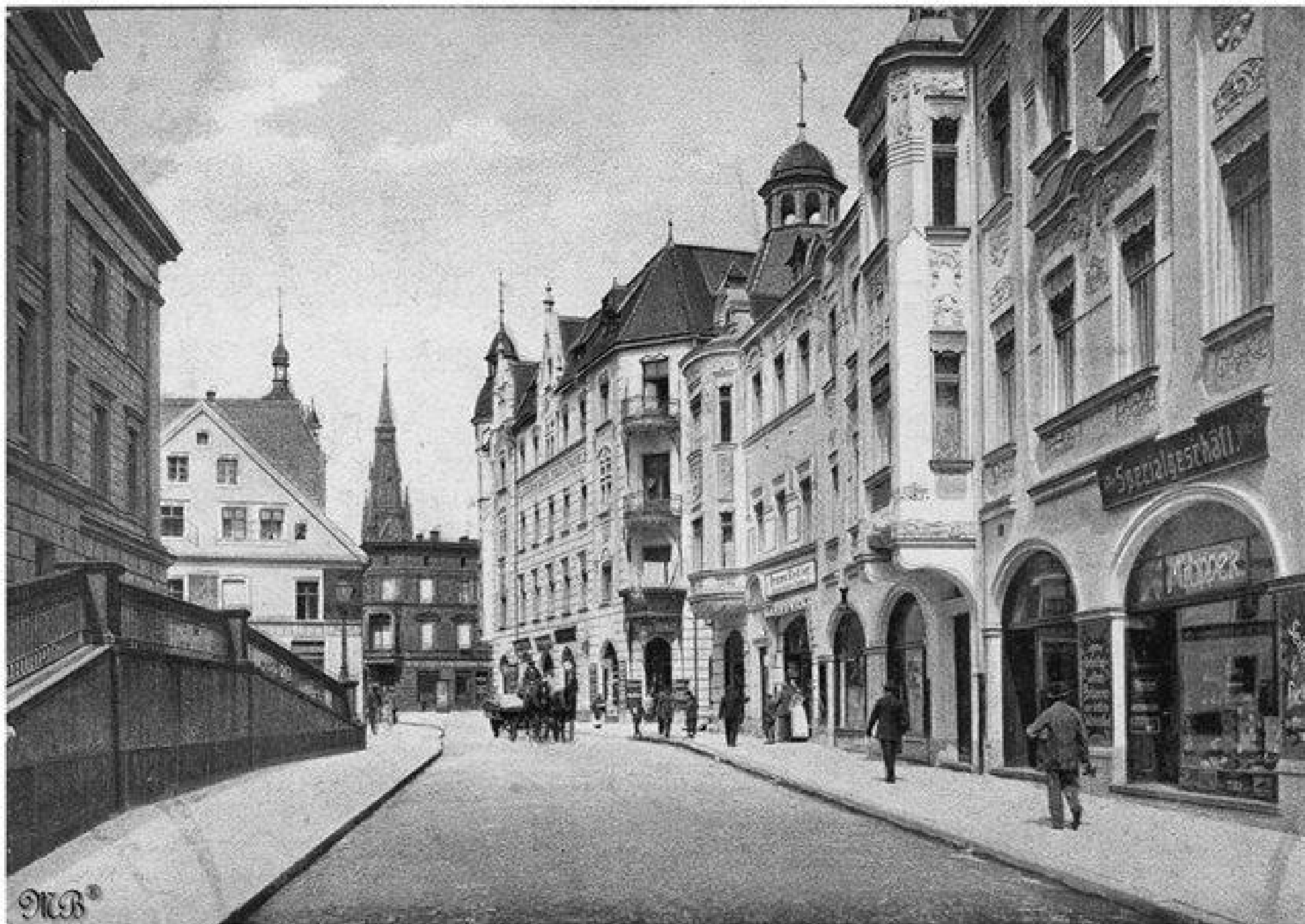
RATIBOR Neue Strasse
